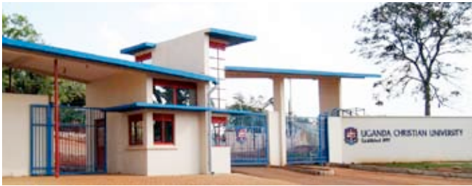
THE UCU CAMPUS' secure entrance gate provides welcome security.
